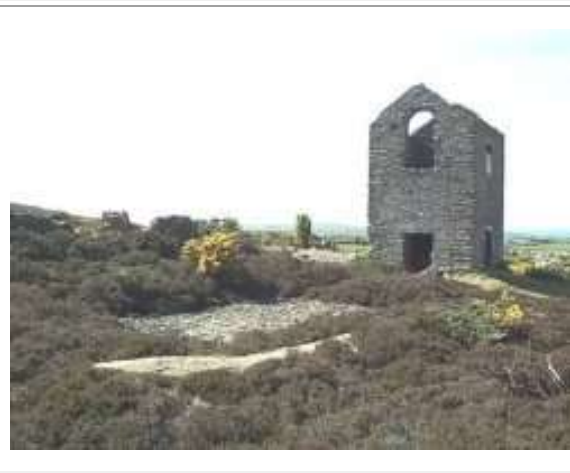
Pearl Engine House 2000
