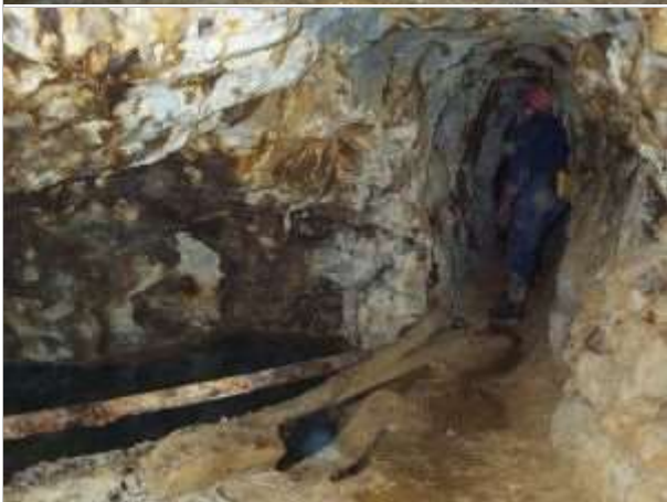
Iron tubes thought to be for carrying compressed air.
