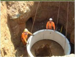
Some of these old air shafts where cleared and made safe. This then allowed the engineers to enter the adit and make a proper assessment of the dam once the water had been removed from the other side of it.
