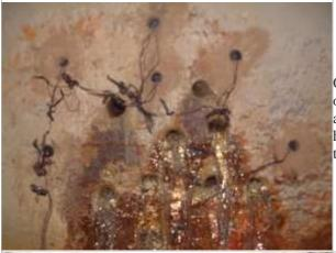
Once safe access to the dam was available a number of test holes were drilled to ensure no significant amount of water was held up behind the dam. A high expansion explosive was then used to destroy the dam.
