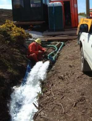
The water was pumped via an existing drainage and settlement system to the Sea at Amlwch Port.
