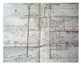
Mona Mines manuscript 3362 is an elaborate Illustration of the levels at Cerrig Y bleddia and Stephens shafts in 1816. Each of these shafts is shown with a horse whimsey in position. Four lower levels are shown for each shaft with the position of ladders and hand whimseys shown.
