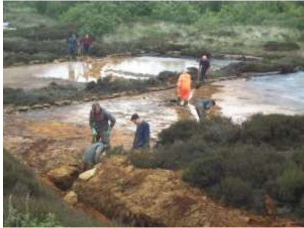
Digging a drainage ditch on the East side of the mountain to drain water from the Dyffryn Coch adit
