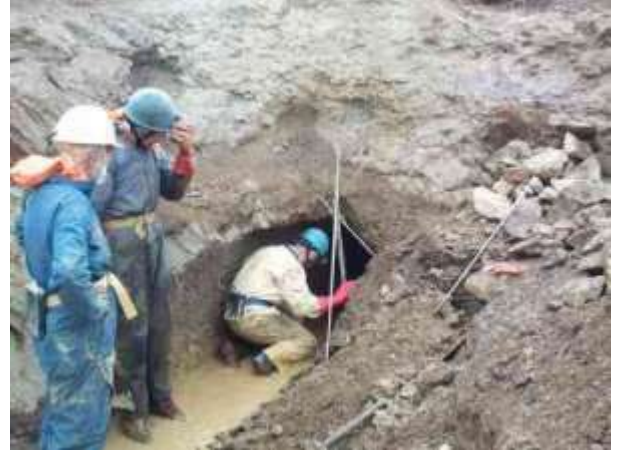
Clearance of the Mona adit drainage ditch. This allowed re-entrance to the adit in early 2000.
