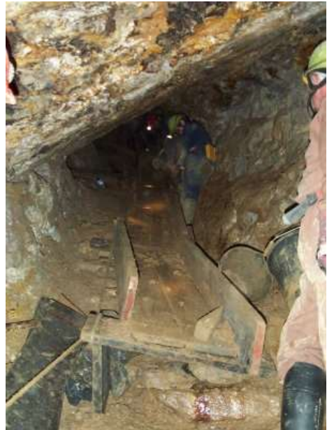
Work on a new Parys mine entrance and the clearance of debris just below ground
