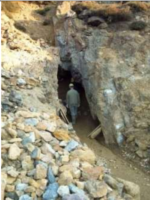
Removal of debris from the Dyffryn Coch adit. This may give access to early 18th century workings
