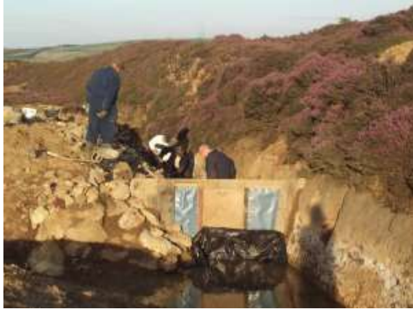
Clearance of the Mona adit drainage ditch. This allowed re-entrance to the adit in early 2000.
