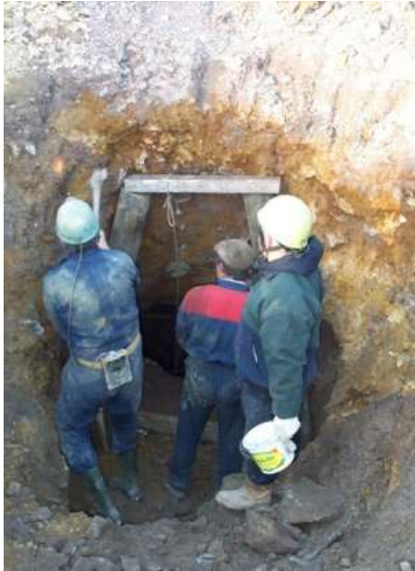
Work on a new Parys mine entrance and the clearance of debris just below ground
