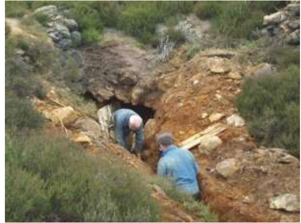
Digging a drainage ditch on the East side of the mountain to drain water from the Dyffryn Coch adit
